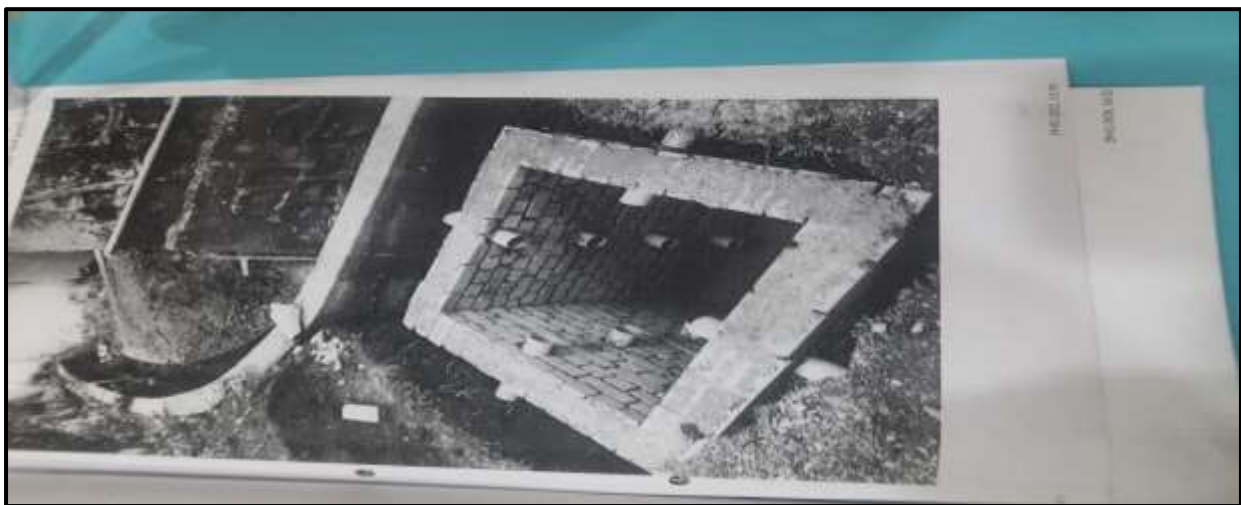
Fig: Pit for rain water harvesting:
